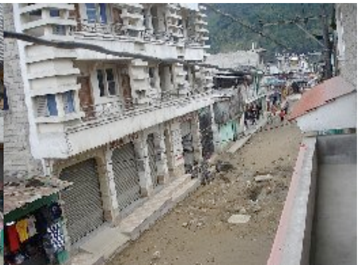
RIGO'S HOTEL IN BARILLAS
